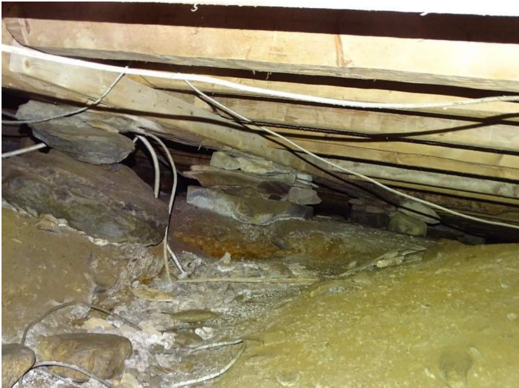
LOWER FLOOR FRAMING AND FAILING PIERS
