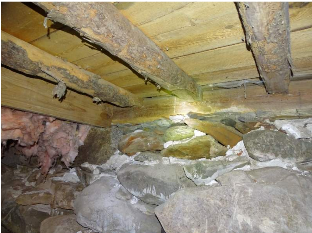
NORTH BASEMENT - SANCTUARY ENTRY FRAMING AND FAILING RETAINING WALL
