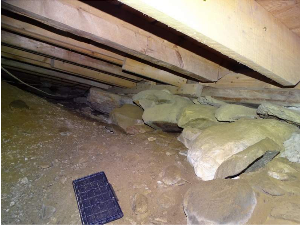
LOWER FLOOR FRAMING AND FAILING FOUNDATIONS
