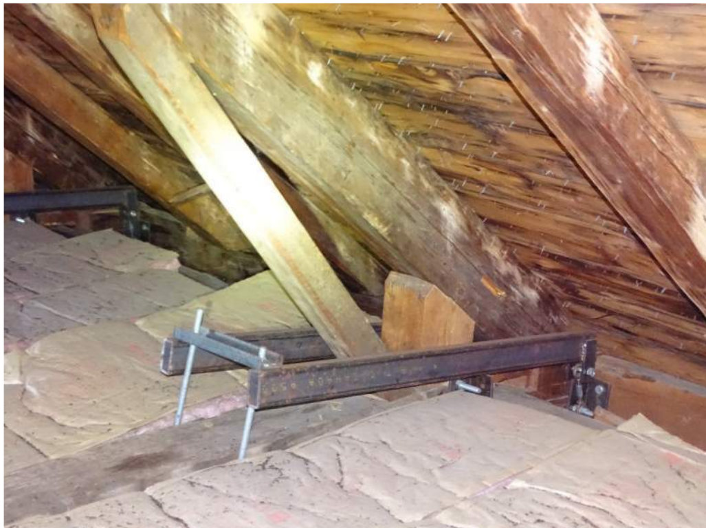
2010 EAVE REPAIR AT TRUSSES
